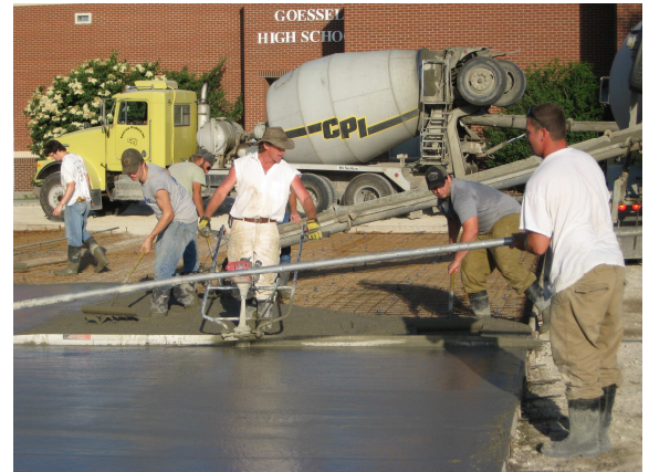
Cement being poured at the HS.
